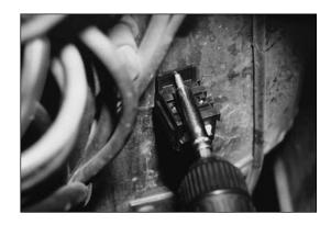
Install the special relay into the receptacle.
