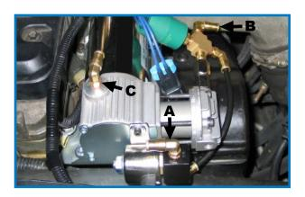
1 1 Consult with the customer for a preferred location for the quick connect airline coupler. Route the supplied airline to this location and connect to the coupler. Connect the other end to the remaining fitting at the compressor head.
